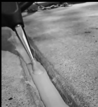
KwixSeal™ Rubber is Applied Hot
